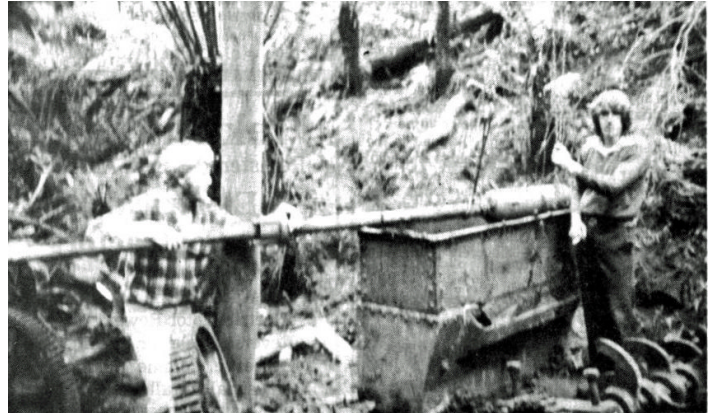
Graham Dyce, supervisor of the project, and Greg Hardy removing stampers to prepare for painting.
