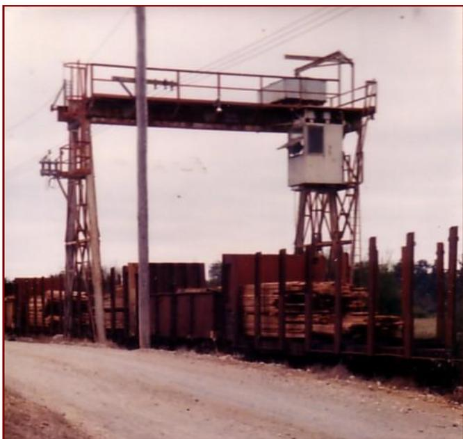
THE GANTRY CRANE — capacity 10 tons
