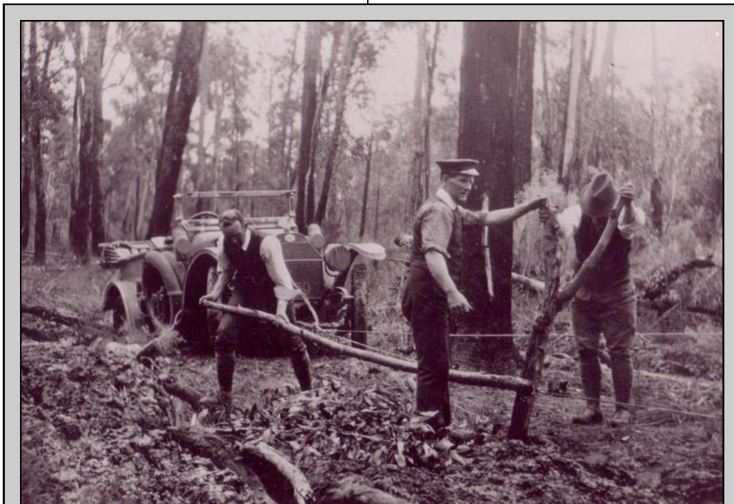
FIG. 2: THE ROAD NEAR HOSPITAL CREEK
