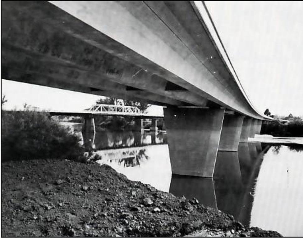
**ABOVE:** *The new bridge — Orbost's fourth since 1891 — dwarfs the old bridge that provided a river crossing for more than 50 years. The new bridge has been built 1.6 metres above the record flood levels of 1971.*
