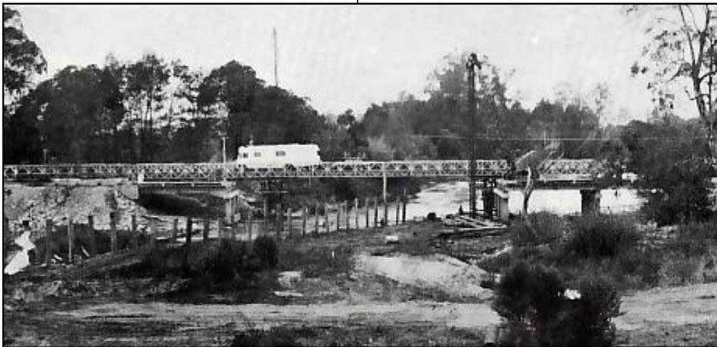
*The old road bridge over the Cann River at Cann River is being removed to make way for a new bridge. A temporary bailey bridge has been erected to carry traffic using the Princes Highway East.*
