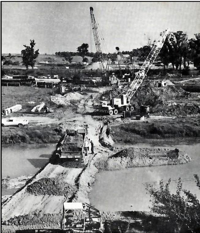
***Pile driving in progress on the east bank of the Snowy River at Orbost. The water in the foreground is a billabong, which, with the main river channel, will be spanned by a bridge 366 metres long.***
