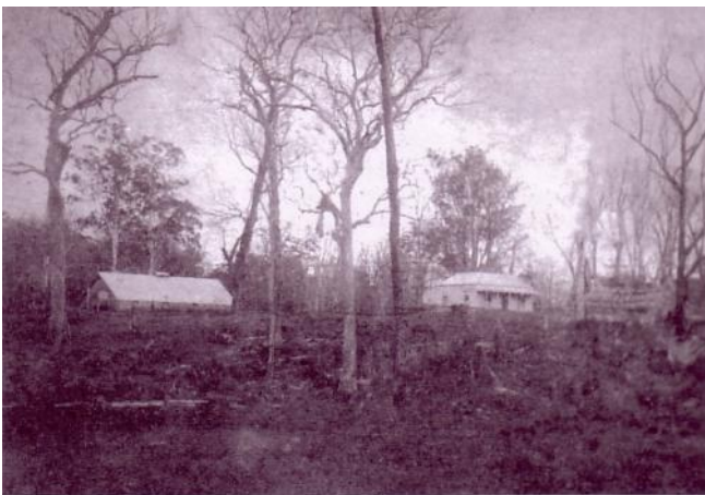
Lochiel Barn and House
