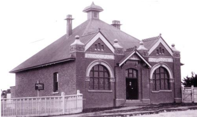
Orbost Shire Council Chambers
