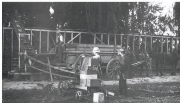
**Maize Elevator designed and built by Percy Watt**
