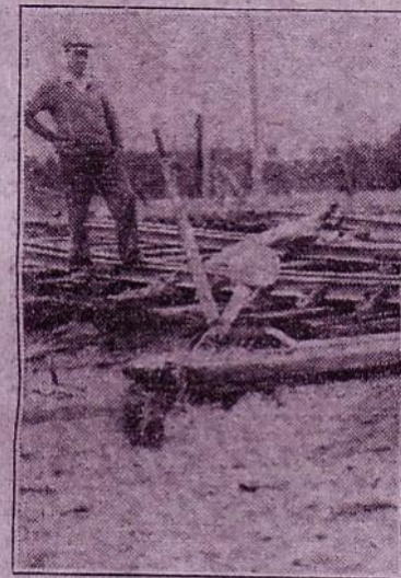
MR. E. NYE, Railways Traffic Inspector in Gippsland, examining the damage done to the permanent way in Orbost station yards.
