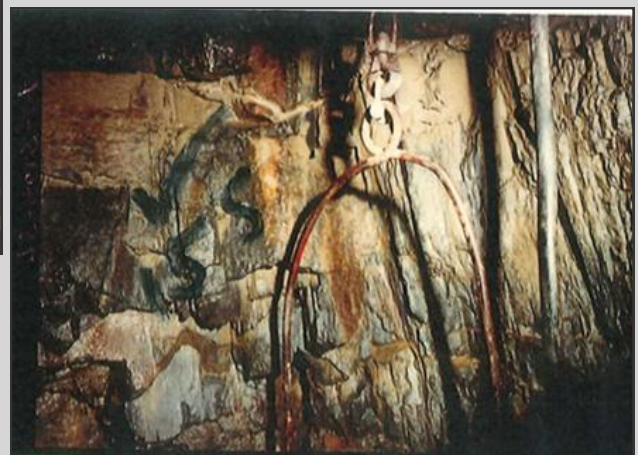
ABOVE: David Jellie about to be lowered inside a steel casing to inspect the rock below. He had to inspect the foundations for each pile.
