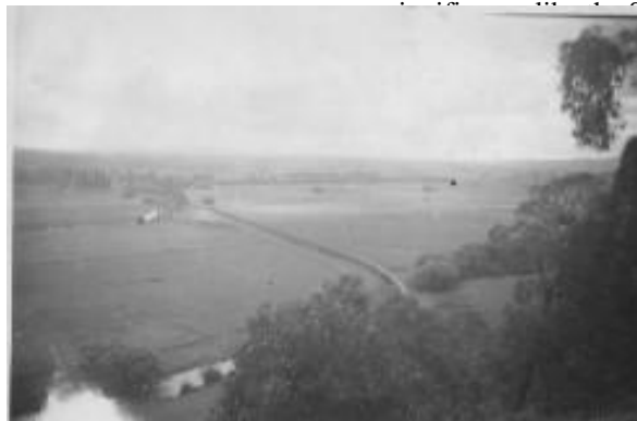
Railway Viaduct across the Snowy River Flats at Orbost
