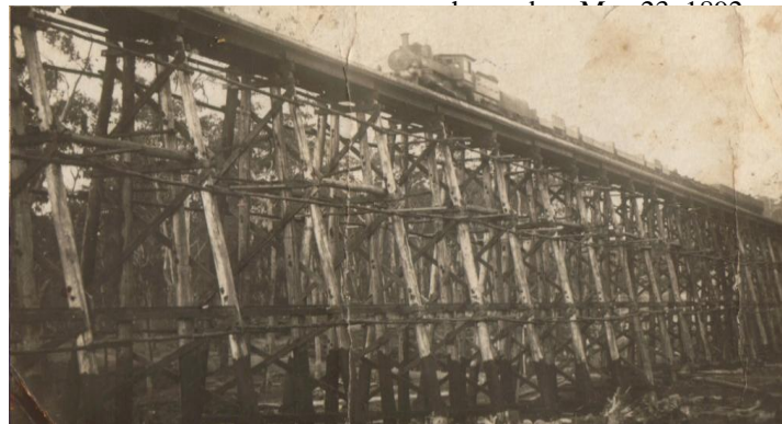
Stoney Creek Railway Bridge west of Nowa Nowa
